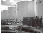
Shock dampening for fuel supply pipings to the aircraft.
